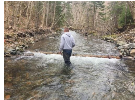
Winter Damage Assessment and Remediation on the Broad Cove River
